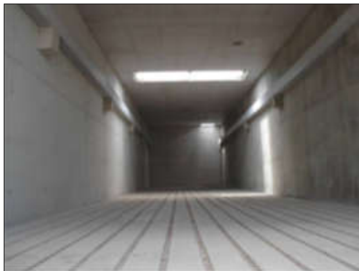
Figure 3-7: Typical composting tunnel with spigot floor
