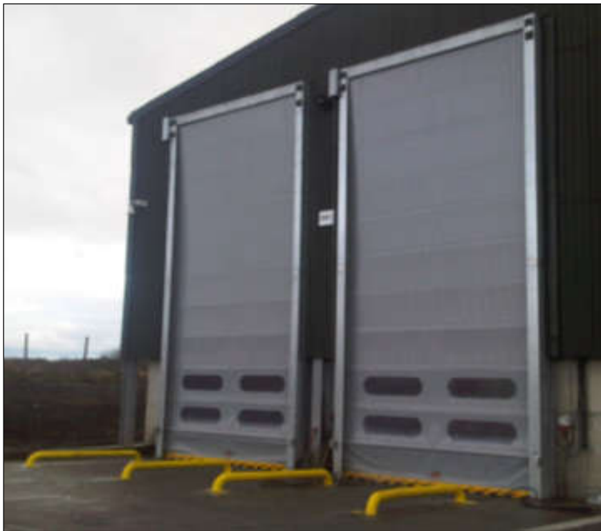
Figure 3-4: Image of waste receiving doors at existing compost plant
